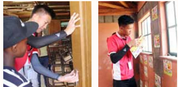
Ernest fixing the door knob for the tribal primary school.
